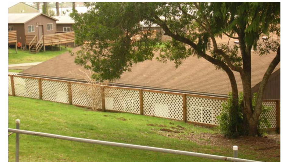
Existing Gymnasium/ Library Building
