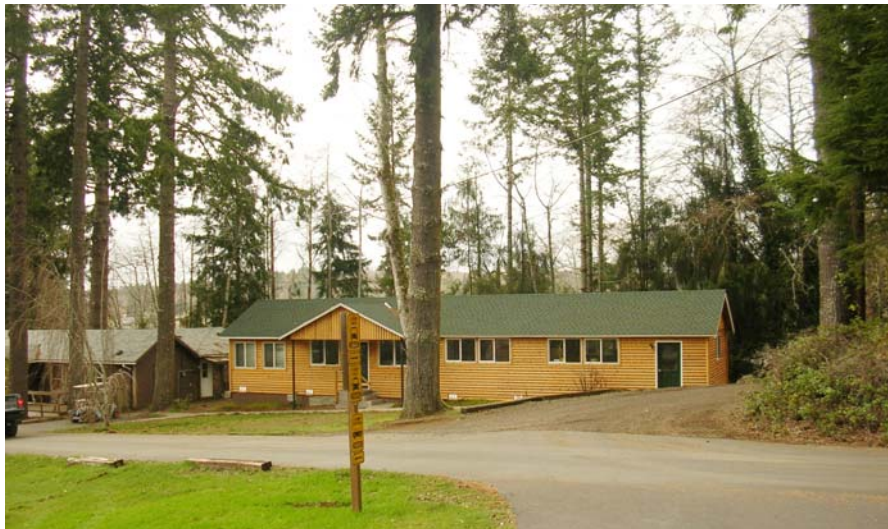
Existing Camp Office and Jewish Enrichment Center
