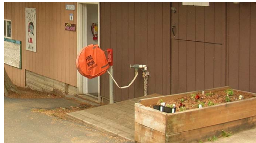
Existing Fire Protection
